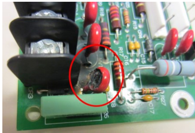
MOVs & Circuit Board Traces Melted
